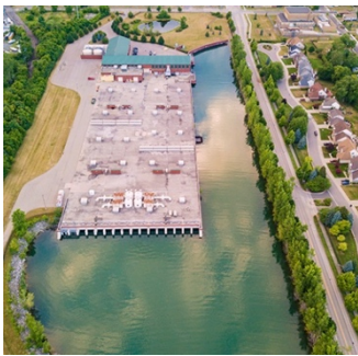
FIGURE 39: CONNER CREEK CSO FACILITY
