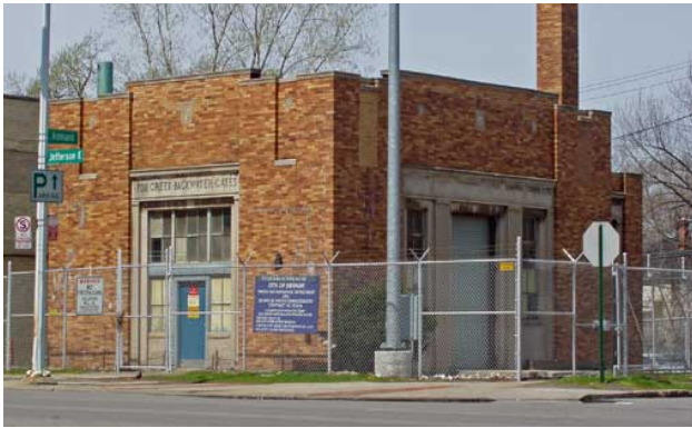
FIGURE 14: HISTORIC FOX CREEK GATES PUMP HOUSE
