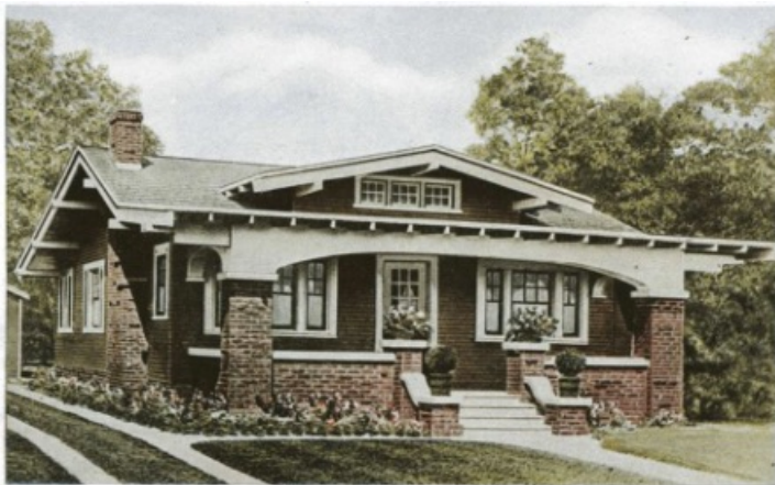
FIGURE 24: TYPICAL ARTS & CRAFTS BUNGALOW AND FOUR SQUARE WITH 5 STAIRS AT 7" TO 8" AN ADDITIONAL STAIR PORCH TO INTO HOME, PLACES THE FIRST FLOOR AT NEARLY 48" ABOVE GRADE
