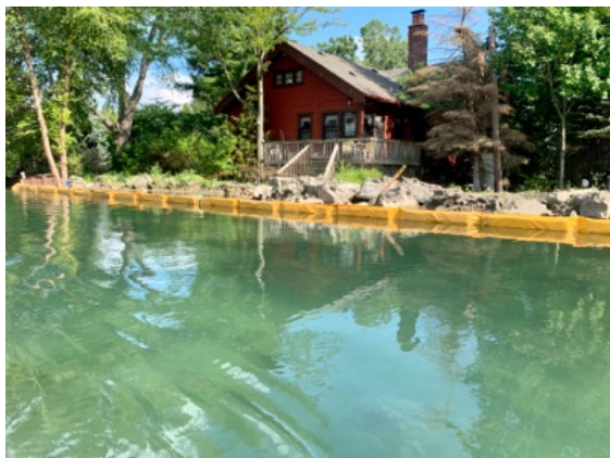
FIGURE 54: PREPARATION FOR SEAWALL
