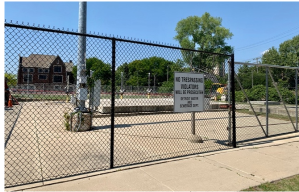
FIGURE 15: CURRENT PUMPS AND EQUIPMENT
