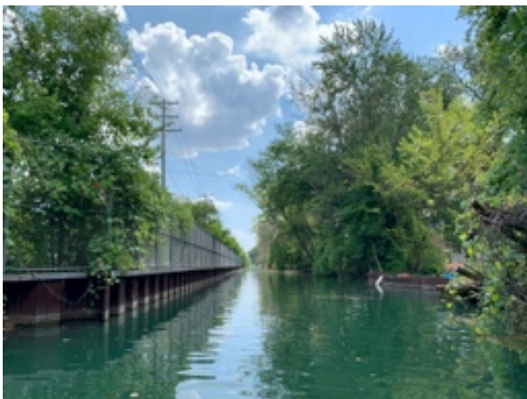
FIGURE 51: ALTER ROAD LEVEE'S EASTERN SEAWALL
